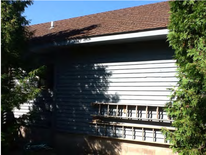
West garage exterior.
